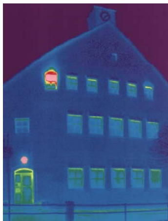
Figure 7: A thermographic picture of the façade from figure 6 after the building's retrofit (the upper left window is tilted).
