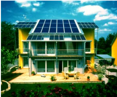
Figure 4: South elevation of a perfectly orientated building. The main glazed façade area faces south and is provided with an overhang that provides shading in summer. Solar panels are also shown, although they are strictly speaking not entirely passive, as they require an electrical pump.
