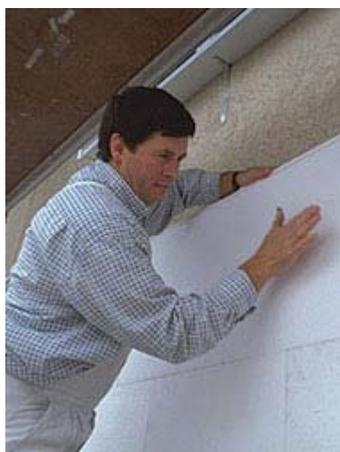
Figure 5: External building shell insulation
