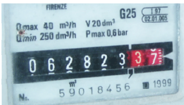
Figure 7: Example of first rough operating energy performance assessment: The reading is 62823 \text{Stm}^3 Installation year is 1999 Reading year was 2006 Yearly consumption was 8974 \text{Stm}^3 per year \approx 86 \text{ MWh/year} Heated surface is \approx 1200 \text{ m}^2 Heating performance is 71,7 \text{kWh/m}^2 per year
